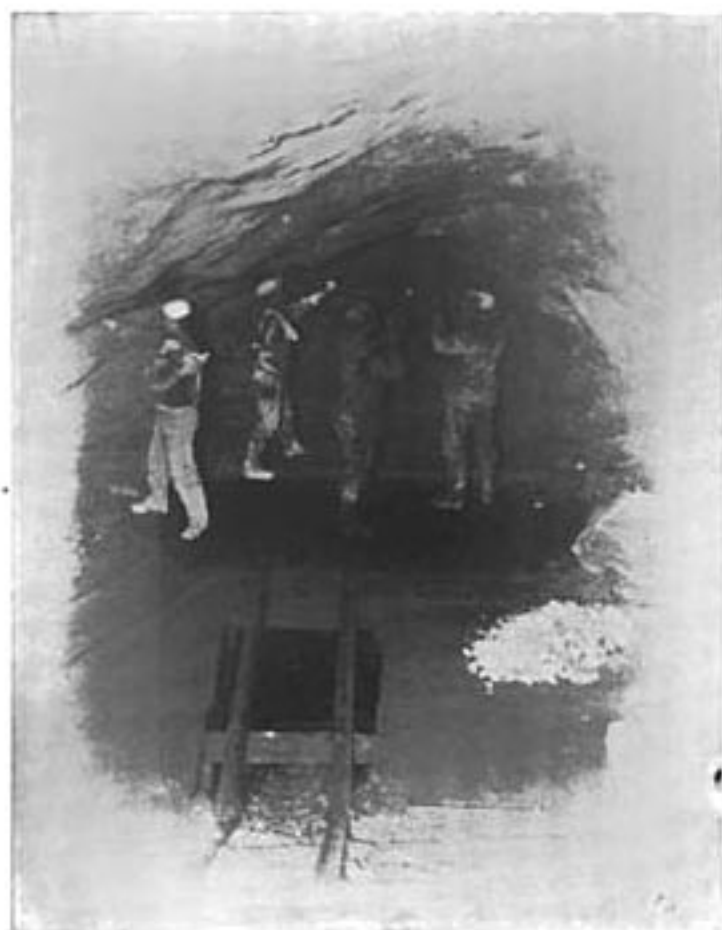
Miners at work Cross-cutting from a Station.
