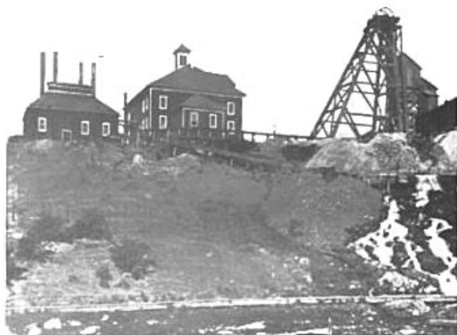
The Cross Hoisting Works.
