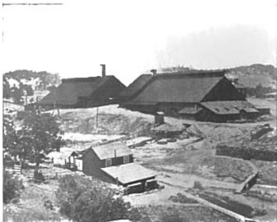
The Chlorination Works.
