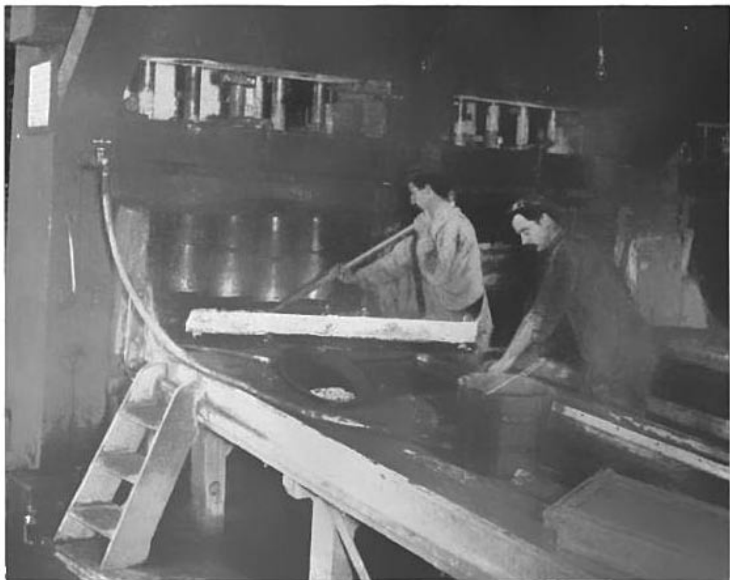
Clean-up of Mill.
