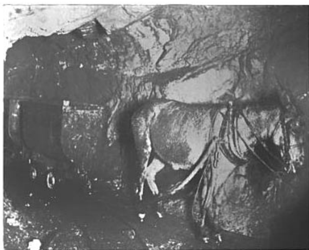
An Ore Train in the Mine.
