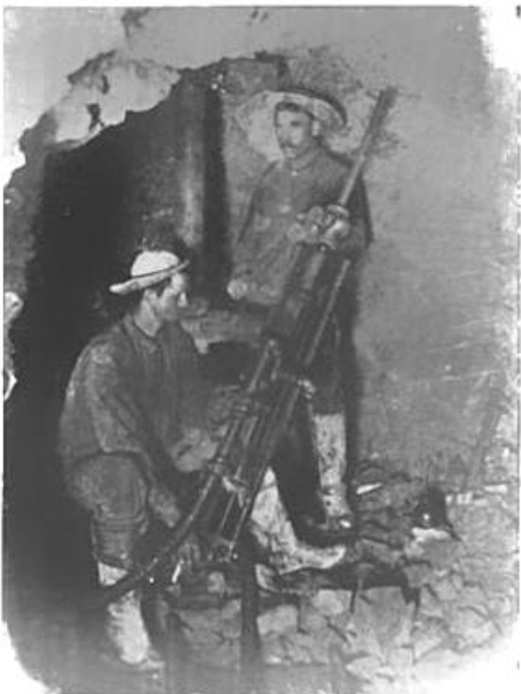
Air-drilling Face of Drift.
