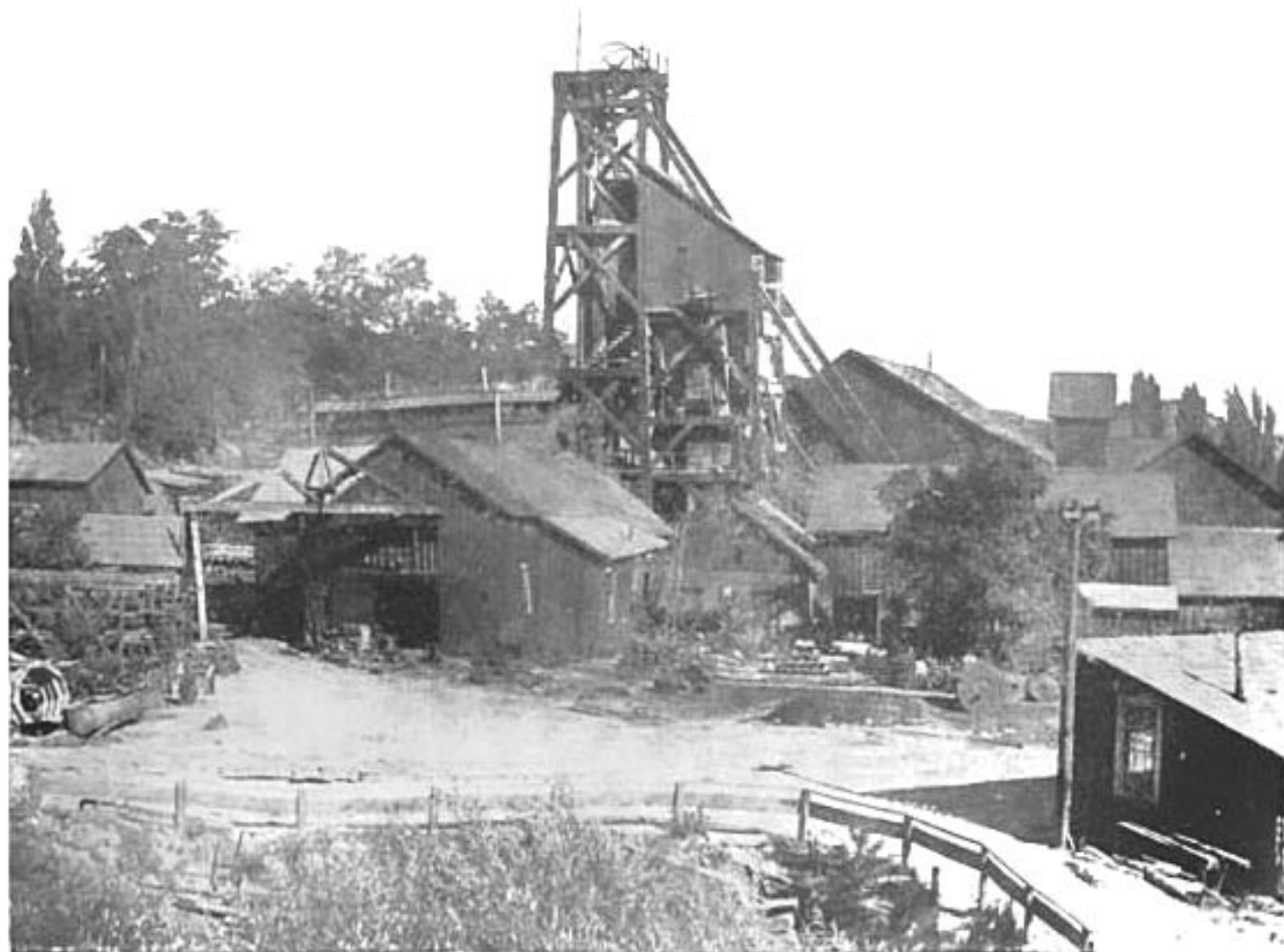
The Sixty-Stamp Utica Hoist and Mill.
