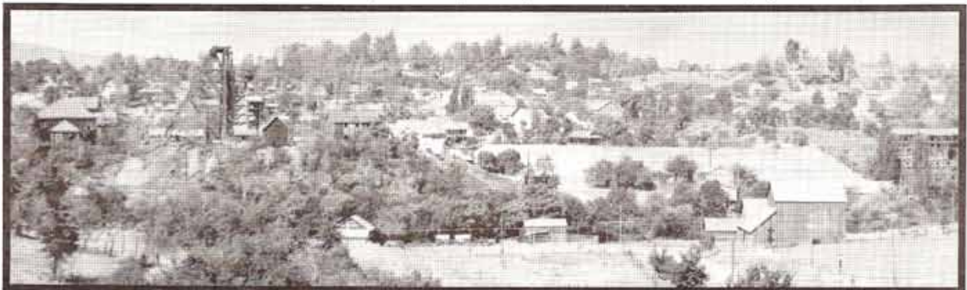
Turn-of-Century Angels Camp was dominated by gold mining operations. At left is headframe of the Utica Gold Mine's cross-shaft with mine dump at center.
